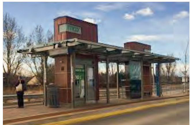
Image 20 – Troutman Station (Built)
